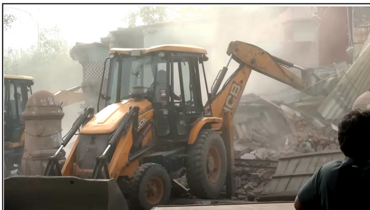
Bulldozers demolishing homes at the Madrasi camp in Delhi in June 2025. Credit: Kritika Pant
